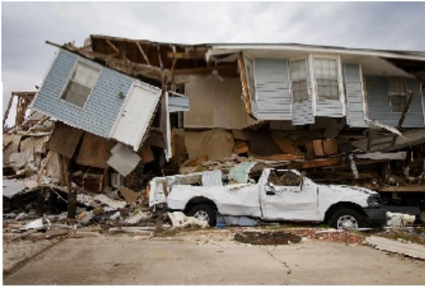
Many homes were completely wrecked
